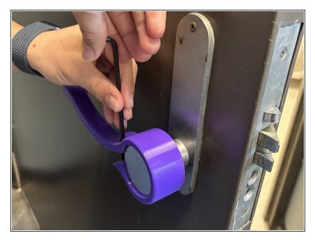
Use the hex key to tighten the bolts as far as they will go to ensure a snug fit
